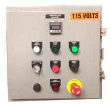
The ETTER Engineering ControlWorx SBCP 1000 is a single burner control panel that provides basic flame supervision to a single gas fired, pilot ignited burner. The High Temperature Limit instrument monitors furnace temperature and will shut down the burner if the measured temperature exceeds the instrument's set-point, as well as setting off an alarm buzzer to annunciate a flame failure.
